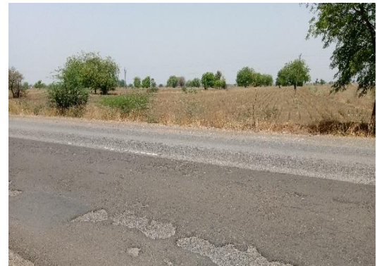
Picture No. 5.1.6: Poorly maintained Wagdhari-Ribbanapalli road (April 2019).
