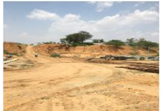
Picture No. 5.1.2: Incomplete bypass at Gowribidanur (May 2019).
